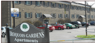
Provide safe, decent, and clean housing.
