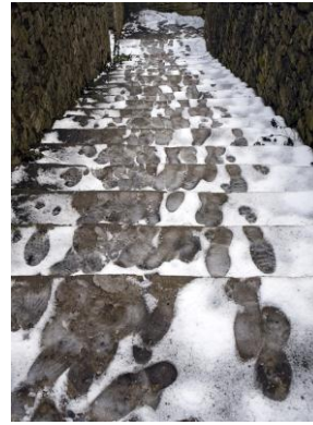
Have slippery steps in cold weather
